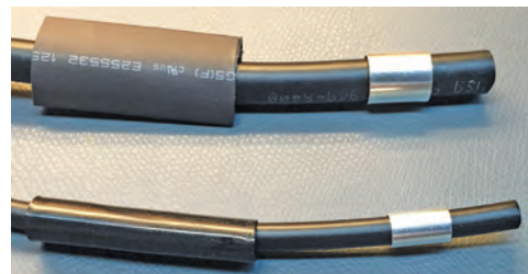
Figure 2 — Start with a square cut across the cable end and slide on the ferrule and a piece of heat-shrink tubing.
